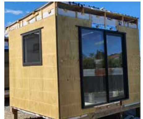
The cabins are taking shape.
